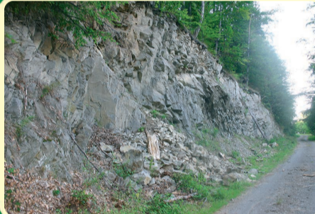
Route between the resting places no. 5 and no. 6
